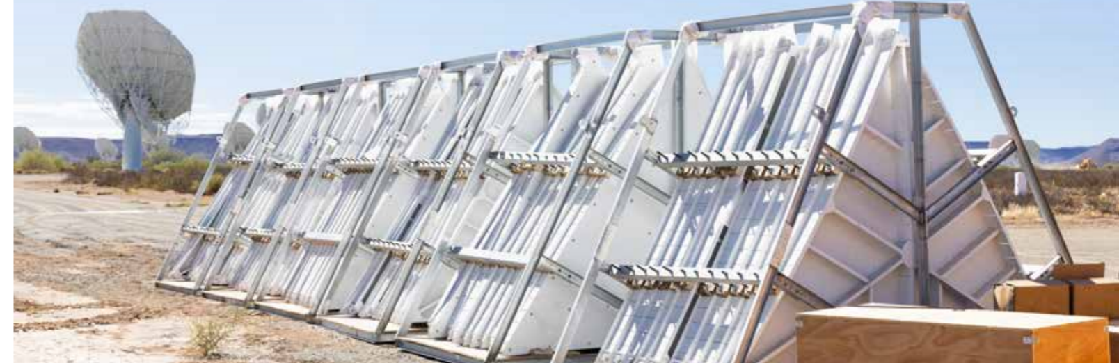
Below: Dish panels on site, waiting to be assembled. Credits: SKAO/SARAO
