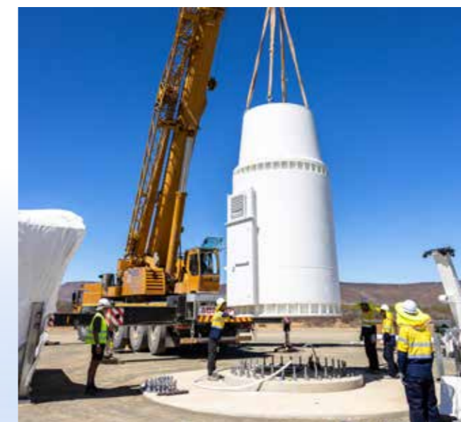
Left: The pedestal is lifted into position.
