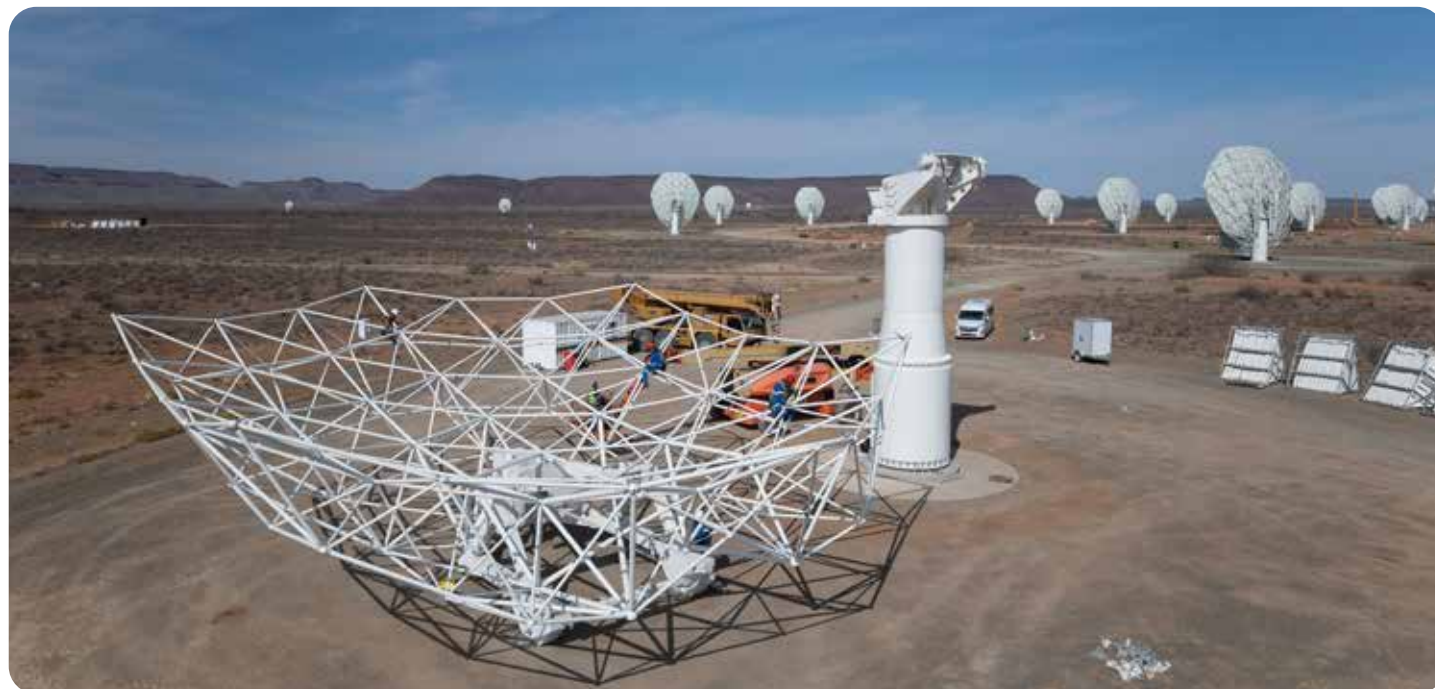
An SKA-Mid dish structure next to its pedestal on the telescope site in the Karoo. Credit: SKAO/Jac Kritzinger
