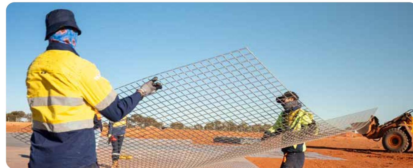
Cape Dunstan contractors lay mesh at the core of the SKA-Low telescope.
