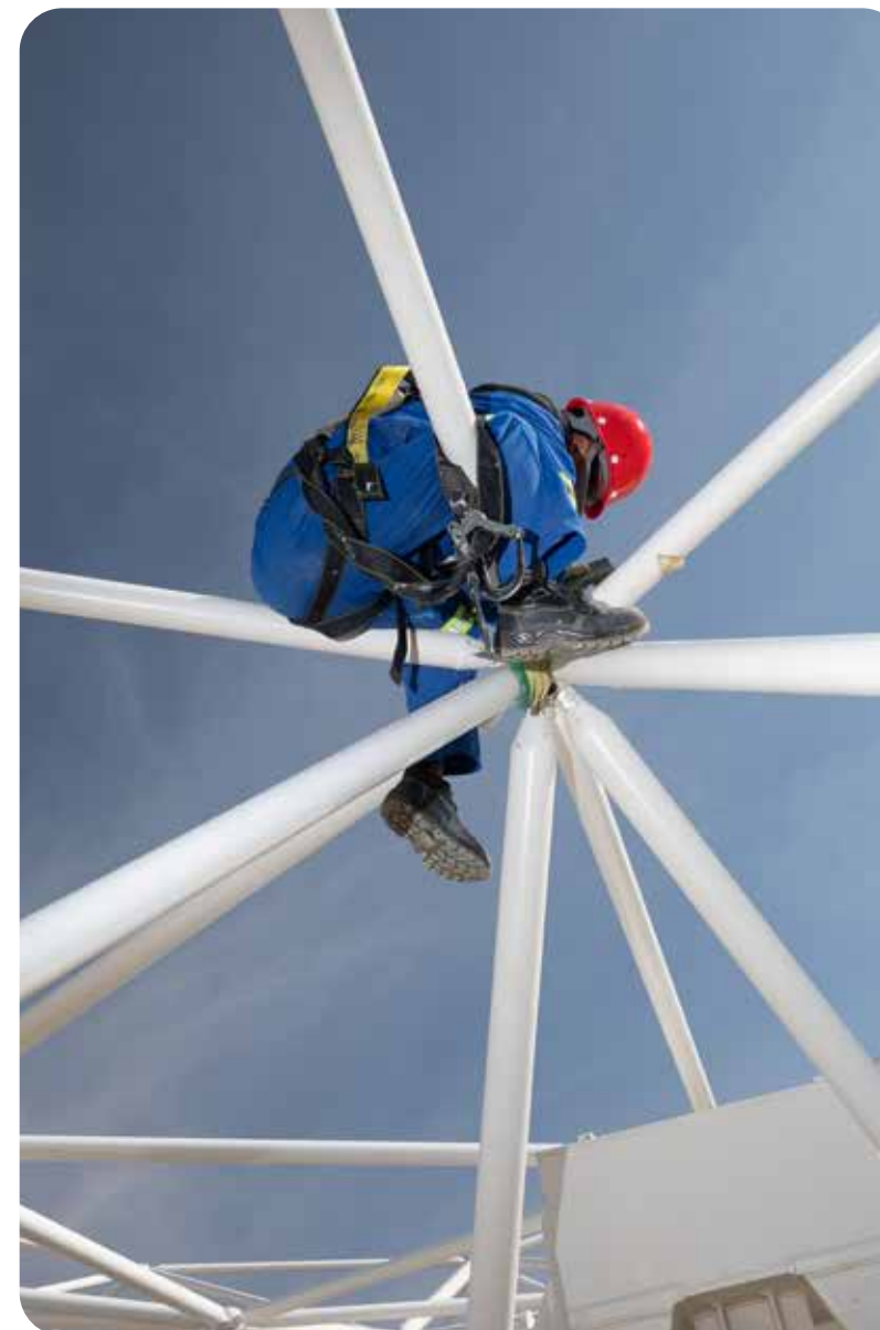
The construction team working on the backup structure of an SKA-Mid dish that will support the 66 panels of the main reflector. Credit: SKAO/Jac Kritzinger
