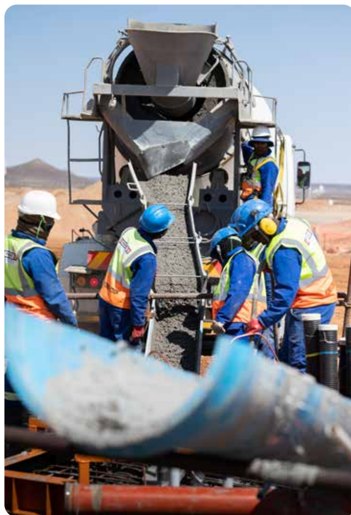
Concrete pouring from a mixer truck into the cylindrical base of an SKA-Mid pedestal. Credit: SKAO/Jac Kritzinger
