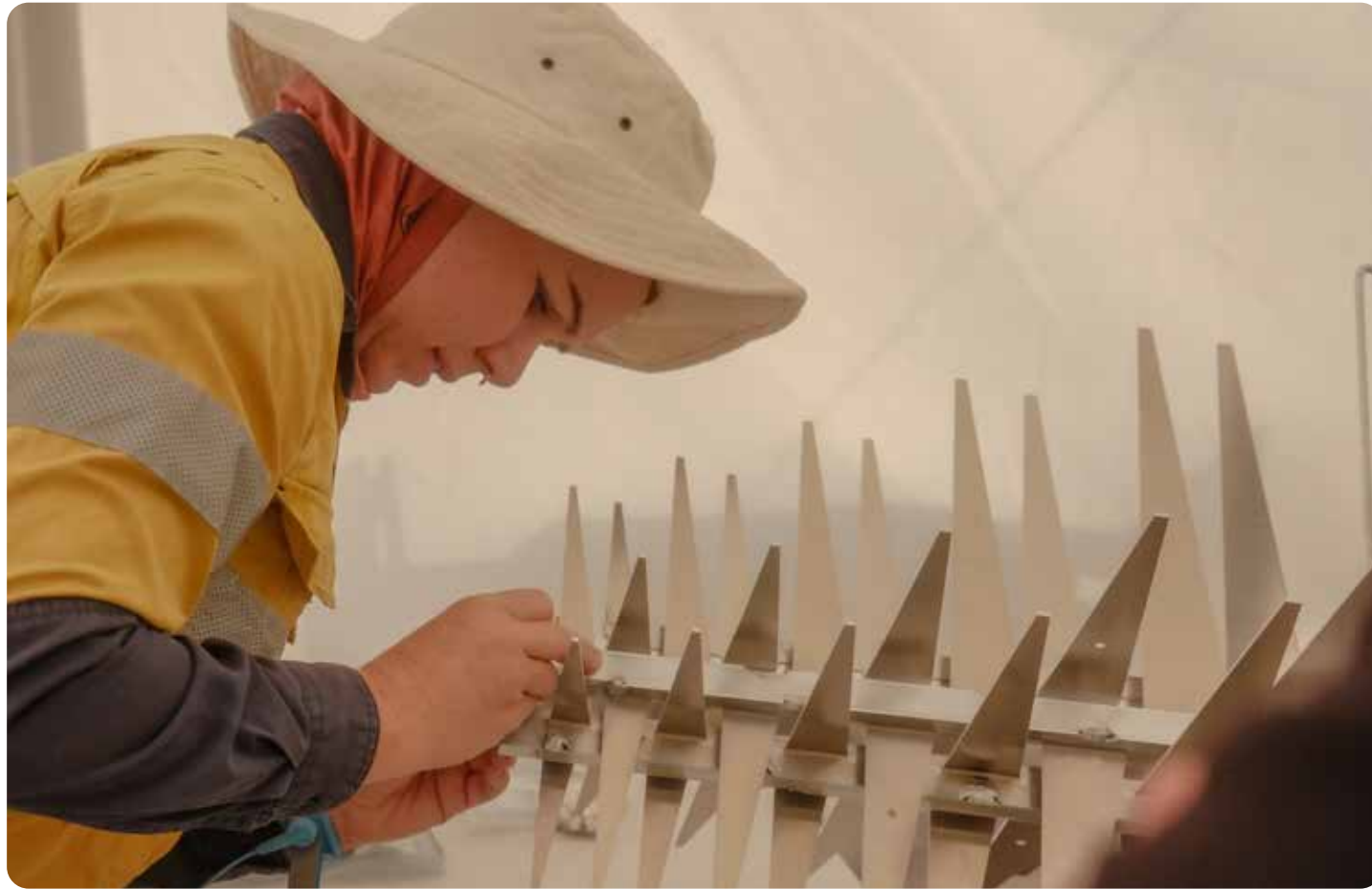
SKA-Low Field Technician Emily Goddard assembling an SKA-Low antenna.
