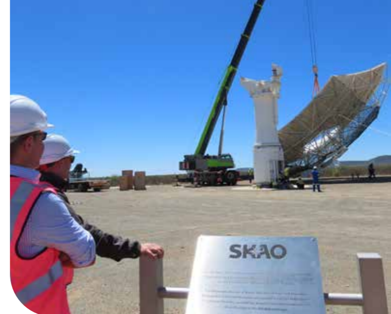
Above: The “big lift” of the second SKA-Mid dish main reflector onto the pedestal on 26 February 2025.
