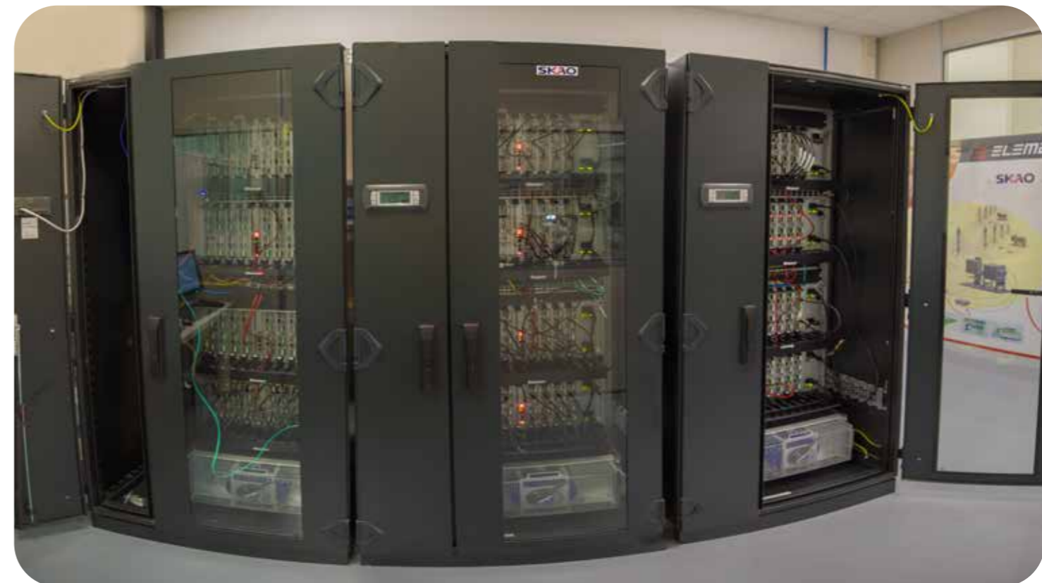
Above: One of the SPS cabinets at Elemaster's SKAO LAB in Osnago. Credit: Elemaster Group
