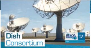
The SKA Dish Consortium is responsible for all activities necessary to prepare for the procurement of the SKA dishes, including the design and verification of the antenna structure, optics, feed suites, receivers, and all supporting systems and infrastructure for SKA1-mid.
